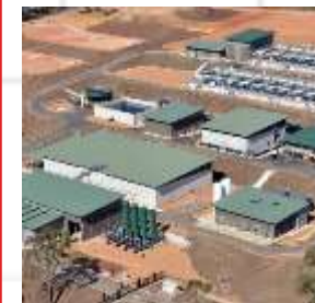
Planta potabilizadora de Mundaring, Perth, Australia
